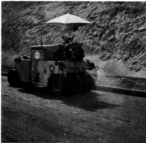
Figure 12. Pneumatic-tired roller on C.T.S. Note fog moisture application.
