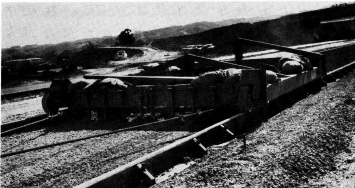
Figure 5. Cement-treated subgrade—windrow machine.
