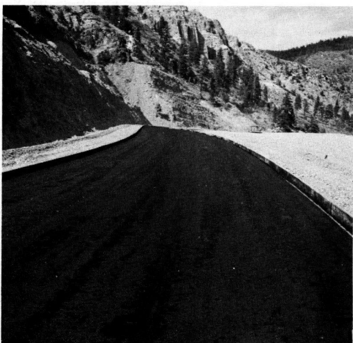
Figure 15. Cement-treated subgrade after application of curing seal.
