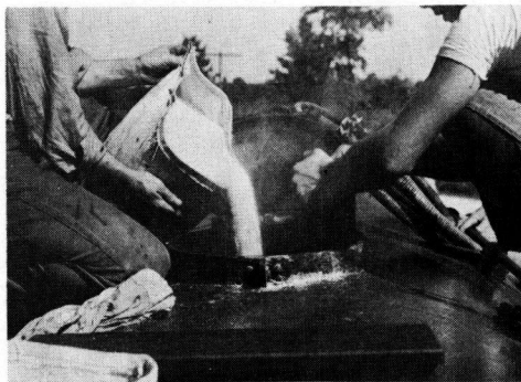
Figure 6. Mixing Powdered Natural Rubber with Asphalt (RC-2) in Distributor - The rubber was added slowly, stirred with a paddle and agitated by the distributor.
