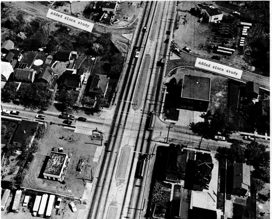
Figure 3. US 1 at Avenel Street, Woodbridge (looking north).
