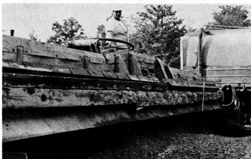
Figure 8. Spreading and striking off concrete with Blaw-Knox spreader.
