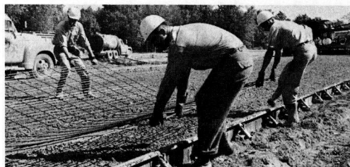
Figure 9. Placing wire mesh reinforcement in continuous section.
