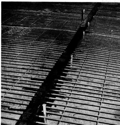
Figure 21. Continuous wire mesh reinforcement in place through joint header.
