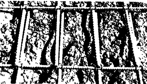
Figure 6. Lap in continuous bar mat reinforcement.
