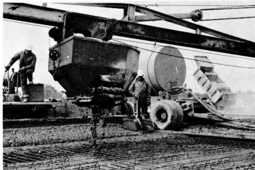
Figure 36. Spreading concrete from bucket behind instrumented standard mesh reinforcement.
