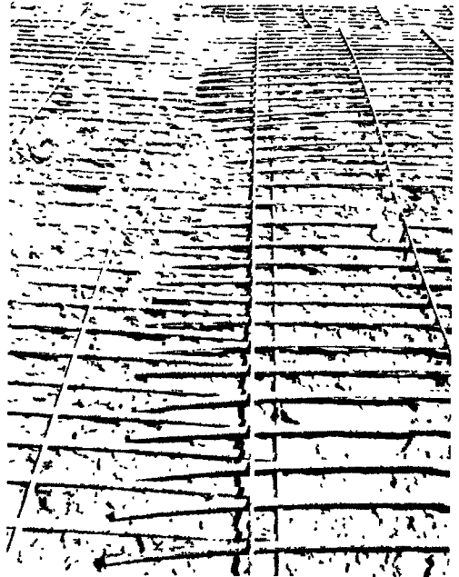
Figure 7. Lap in continuous wire mesh reinforcement.
