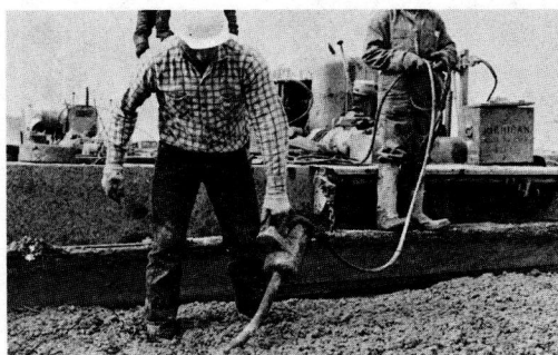
Figure 39. Vibrating concrete adjacent to instrumented standard mesh reinforcement.
