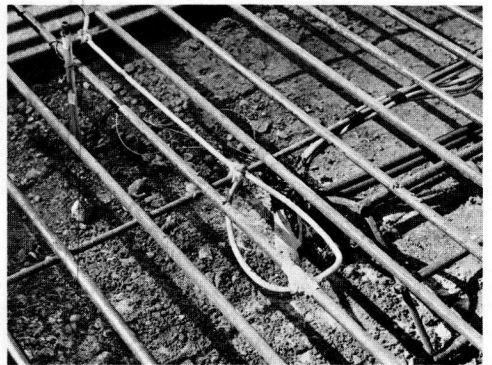
Figure 34. Instrumented wire mesh reinforcement with corrugated crack former and thermocouples.
