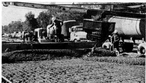
Figure 11. Placing final layer of concrete on bar mat reinforcement.
