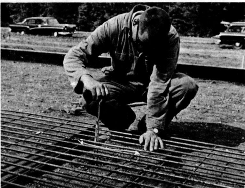
Figure 33. Placing plastic tube containing thermocouples in subbase.
