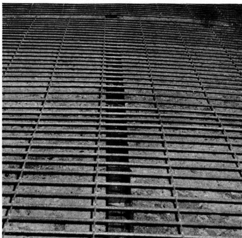
Figure 19. Continuous wire mesh reinforcement placed over lower set of 4 by 4's.
