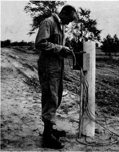
Figure 40. Wiring strain gage and thermocouple leads at junction box.
