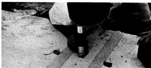
Figure 46. Measuring surface crack opening with graduated scale microscope.
