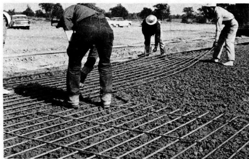
Figure 10. Placing bar mat reinforcement in continuous section.
