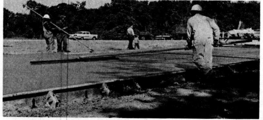
Figure 15. Final hand finishing of concrete surface.
