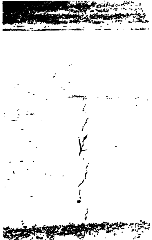
Figure 9. Typical transverse crack in non-reinforced pavement. Crack open \frac{3}{16} in. in 30-ft panel. Division 1, Sta. 220 + 93.
