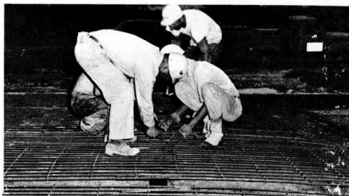
Figure 20. Wiring dowel bars to wire mesh reinforcement.
