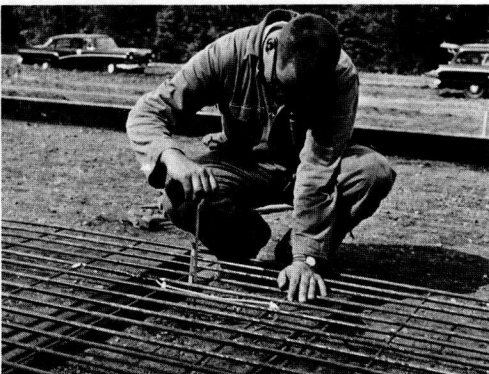
Figure 33. Placing plastic tube containing thermocouples in subbase.
