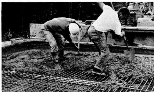
Figure 37. Placing concrete around corrugated crack former in heavy mesh reinforcement.
