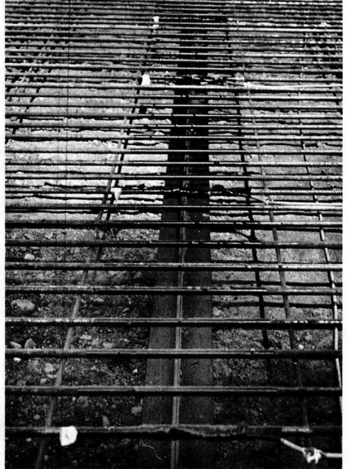
Figure 32. Instrumented wire mesh reinforcement in place.
