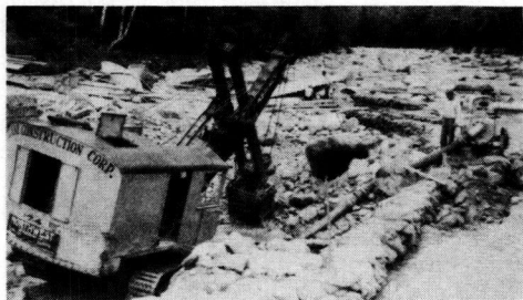
Figure 11. View Showing Tightly Cemented Boulder Formation Predicted from Seismic Tests at Pemigewasset River Crossing Near Lincoln, New Hampshire
