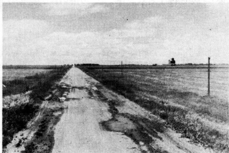
Figure 25. Poor Highway Performance on Glacial Lakebed Soils of Ward County, North Dakota
