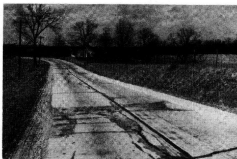
Figure 13. Concrete Pavement in Central Lawrence County, Indiana - Pavements often break up in shallow road cuts in the clays of limestone regions.
