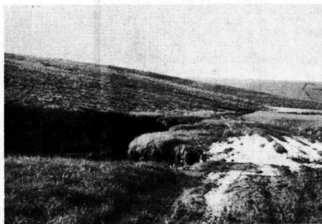
Figure 18. An Illustration of a Severe Thaw in a Local Valley Fill Situation Resulting from Excessive Flow of Water in a Gully Near the Edge of the Road
