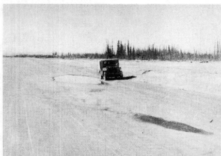
Figure 2. This shows a severe settlement in an airfield runway surface which resulted from thawing subgrade soils.
