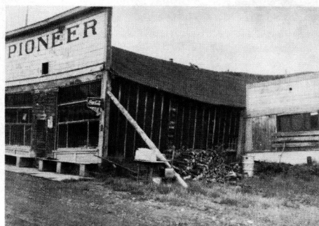
Figure 3. Note the general warping of this building situated on frozen silt which has thawed considerably. The support indicates the severity of the situation.
