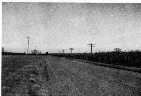
Figure 23. Flexible Pavement Constructed on an Ohio River Granular Terrace, Switzerland County, Indiana (20) - Only very shallow side ditches are required because of good internal drainage of the terrace materials. Highways on granular terraces usually give excellent performance.
