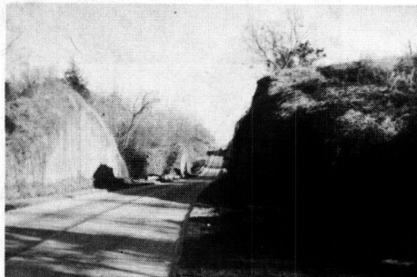
Figure 34. Highway Constructed Through Ridges of Loess, North of Vicksburg, Mississippi - Road cuts are vertical.
