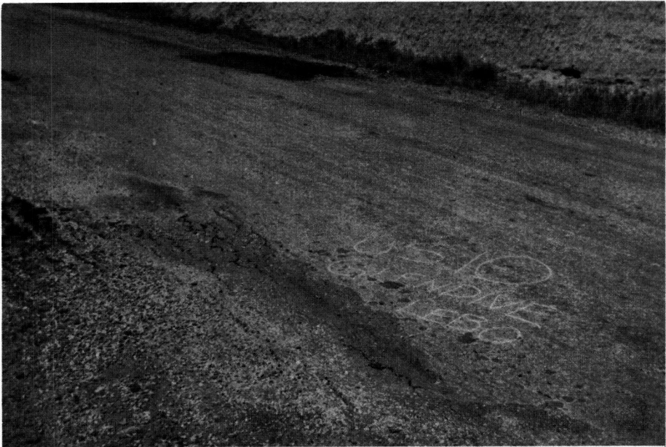
Figure 15. Poor Performance of Flexible Pavement Constructed on Clay Shales of the Northern Great Plains, Near Glendive, Montana - Lebo shales are similar to those illustrated in Figure 14.
