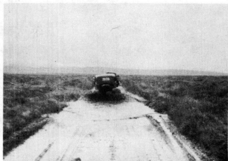
Figure 1. This is a picture of a highway which was constructed on frozen silt which contains pockets of ice in wedge form. The ice has thawed and considerable settlement has resulted as indicated by the deep water puddle.
