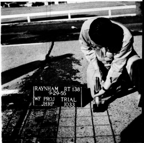
Figure 10. Remington stud driver used to hold down fabric sheets.
