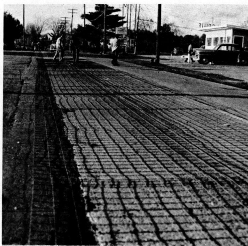
Figure 12. Placing continuous sheet reinforcing.
