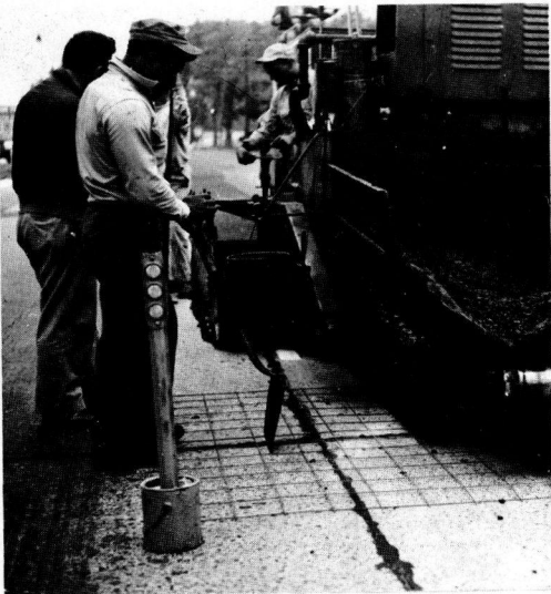
Figure 9. Typical installation of transverse reinforcing over joint.
