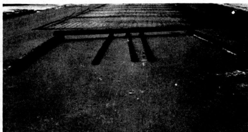
Figure 14. Sled used on Barber-Greene paver for holding down continuous reinforcing.
