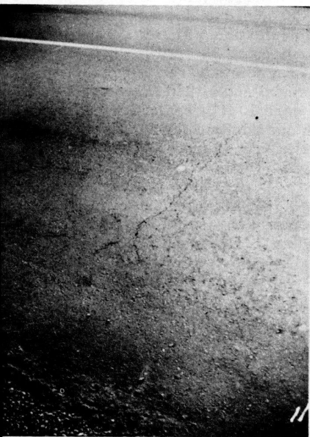
Figure 5. Typical transverse and widening cracks, Sta. 120 to 130.
