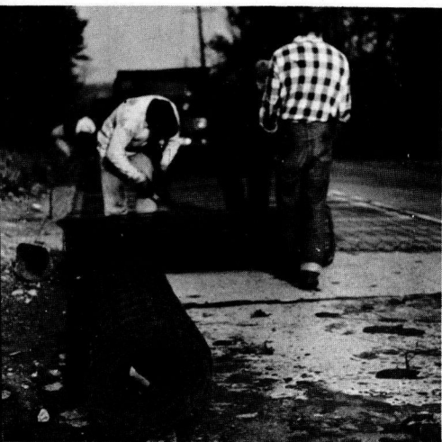
Figure 13. Placing continuous roll reinforcing.
