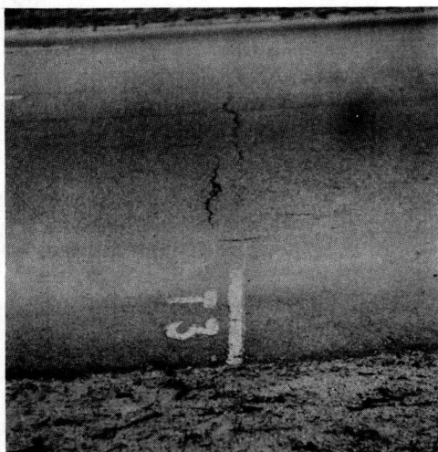
Figure 16. Crack above joint in reinforced section, Raynham.
