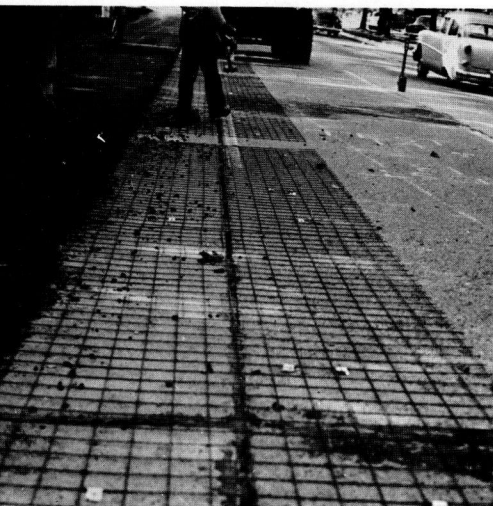
Figure 11. Typical installation of longitudinal reinforcing over joint.
