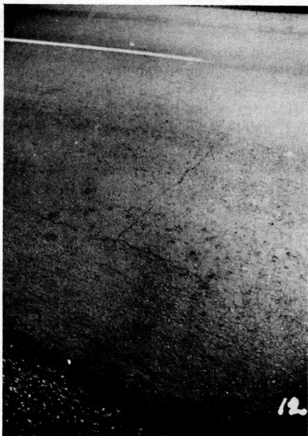
Figure 5. Typical transverse and widening cracks, Sta. 120 to 130.
