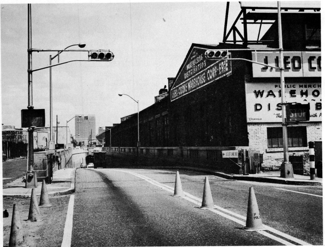
Figure 19. Entrance traffic signals.
