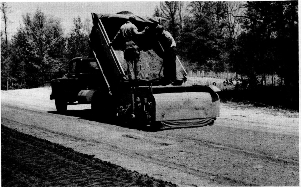
Figure 94. Mechanical cement spreader delivering flat spread for flat-type mixing equipment.
