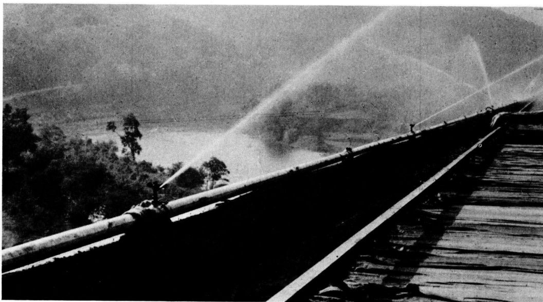
Figure 10. When wet burlap is used for curing it must be kept saturated.
