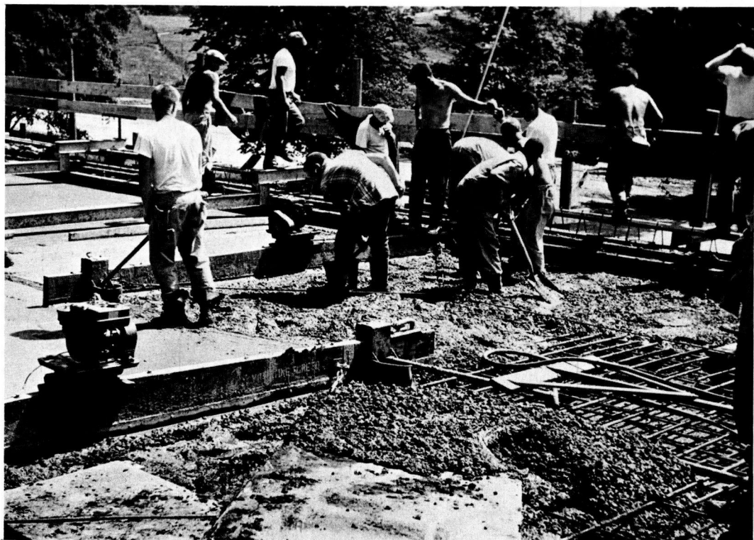
Figure 5. Finishing machines or vibrating screeds should move at a uniform rate and strike off the full paving width in one operation.
