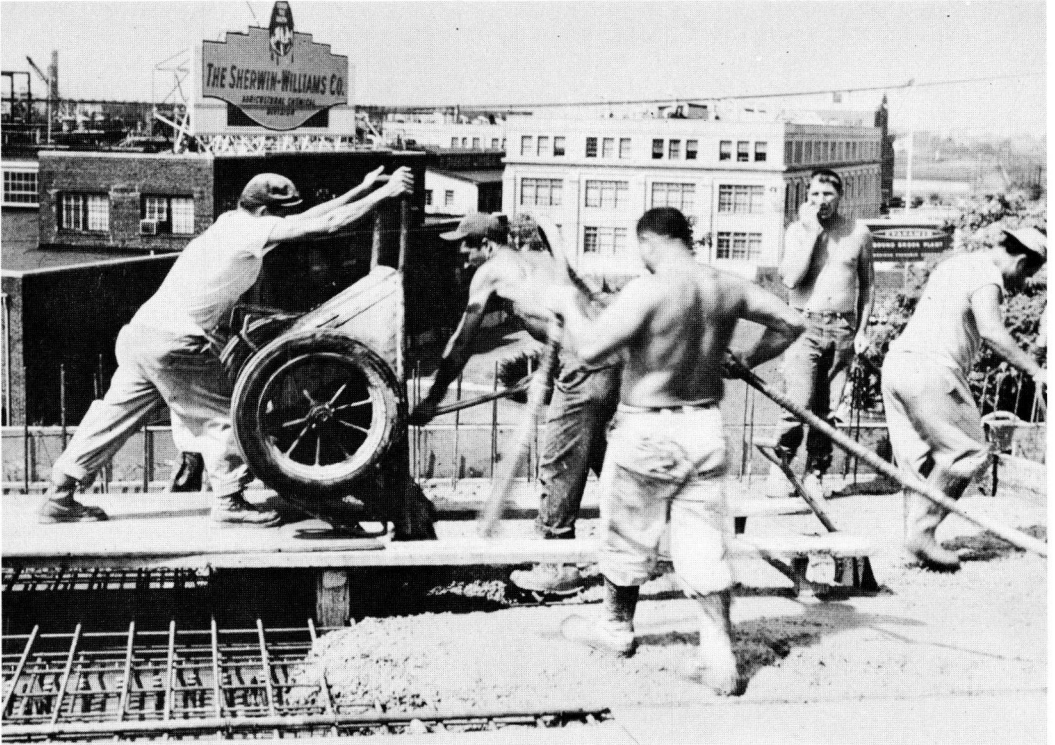
Figure 4. Concrete should be workable and have a 2- to 4-in. slump. Concrete should be placed against concrete and as near its final position as possible.
