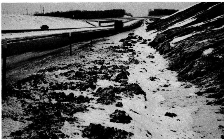
Figure 18. View showing heaving of the ditch, shoulder, and outer pavement lane.
