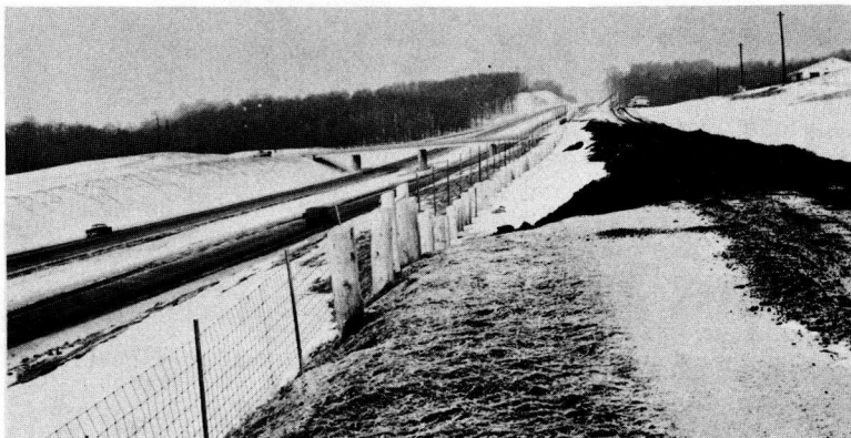
Figure 17. Sag at top of slope, shown by drop of guard rail posts.
