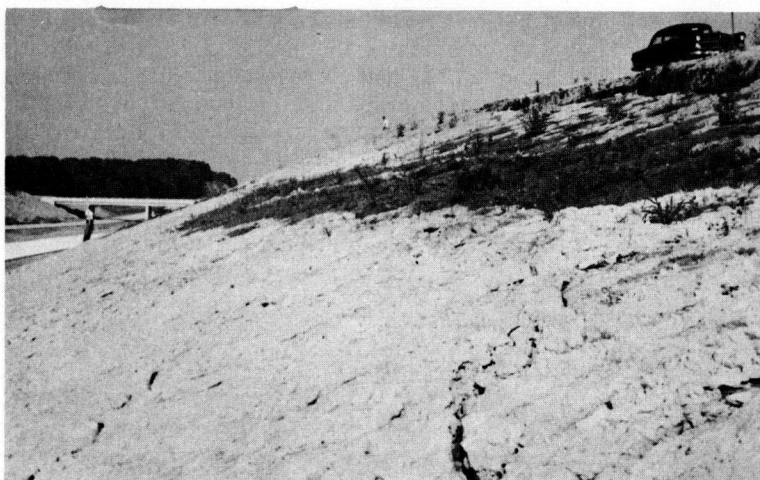
Figure 14. Diagonal tension cracks in the mid-portion and upper portion of the slope.
