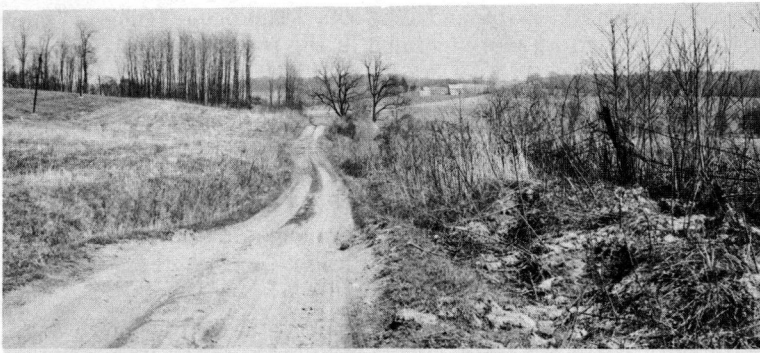
Figure 5. This farm drive, prior to construction, is located at about the top of the proposed cut slope. Note sag in topography, and direction of surface drainage along gentle slope from left to right.
