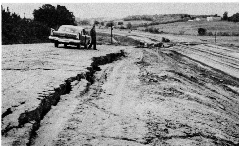
Figure 12. Crack at top of slope, indicating slope failure.
