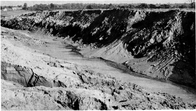
Figure 8. Deep side ditch maintained through cut during excavation, showing erosion.
