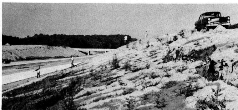
Figure 15. Cracks and downward displacement of intermediate soil mass.
