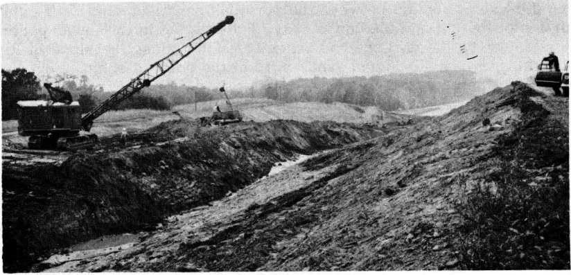
Figure 7. Excavating soft wet soil by using drag line working on mats.
