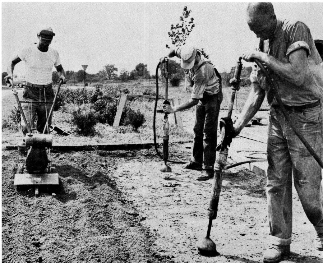
Figure 7. Mixing and compacting treated soil at Creve Coeur, Mo., August 1958.
