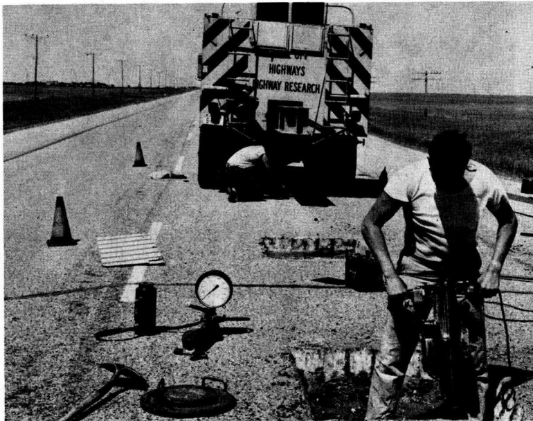
Figure 7. Loosening base course.
