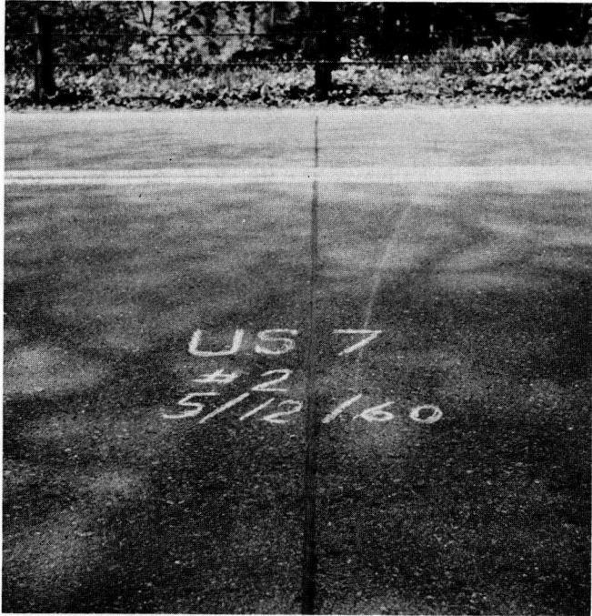
Figure 3. Controlled Joint Crack Project No. 1—Route US 7, Norwalk, May 12, 1960.
