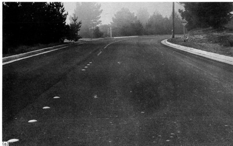
Figure 4. Daytime views of test section on Skyline Boulevard. (a) Inconspicuous curb lights mounted on both sides of test section near Bacon Road. There is a gap in light pattern at curve. (b) Straight portion of test section seen from curve shown in (a).
