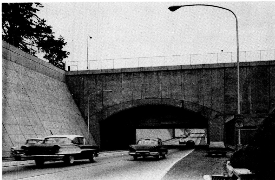
Figure 3. Kingston, N.Y., Intersection entry to New York Thruway arterial spur; illumination at intersection, 3 to 4 ft-c; approaches, 3 ft-c.
