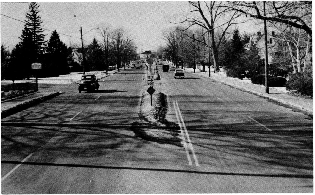
Figure 8. Control Section 40—median openings.
