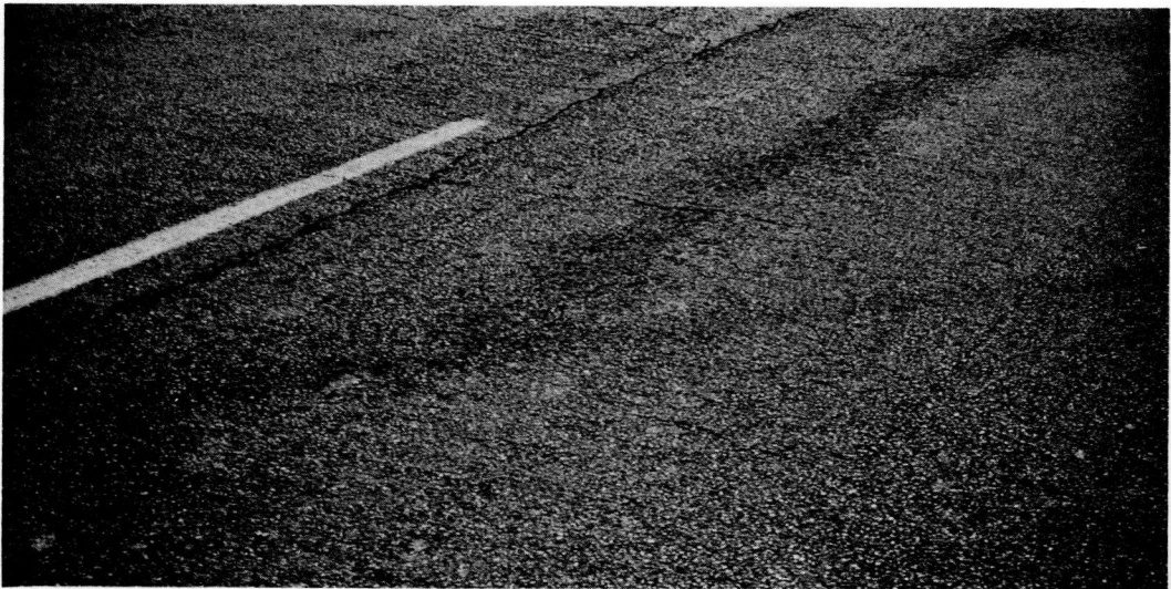
Figure 10. Garrard County SP Group 16 test section (October 1961). Note rough, open texture and pronounced center joint.
