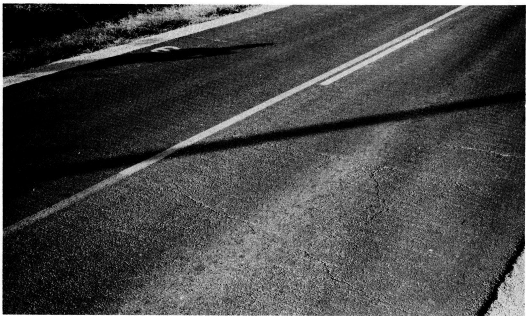
Figure 6. Transverse cracks reflecting through Curtiss-Wright binder mix near station 370 of Nelson County SP Group 31 (one year after surfacing).
