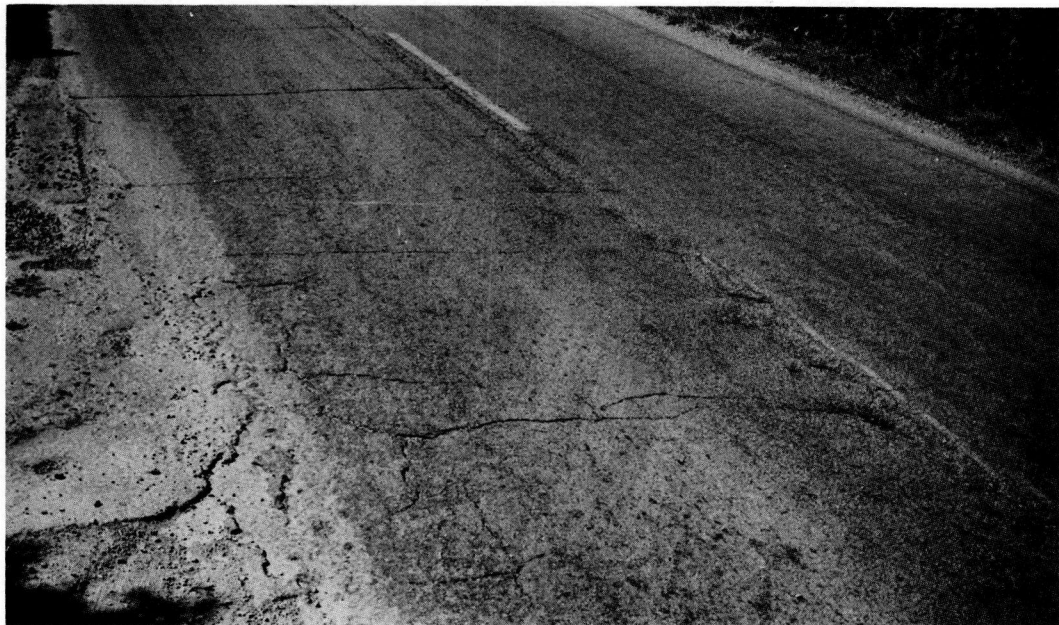
Figure 5. Area of transverse cracking near station 370 of Nelson County SP Group 31 test section (before surfacing with Curtiss-Wright binder).
