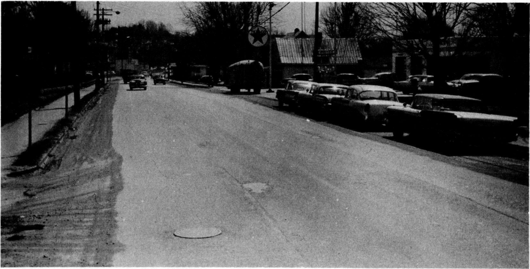
Figure 9. Raveled area near middle of SP Group 11, Laurel County urban test section (6 months after paving).
