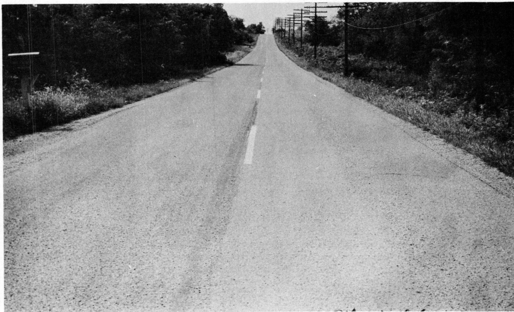
Figure 7. Nelson County SP Group 31 test section after an asphaltic emulsion seal coat had been placed (October 1961).
