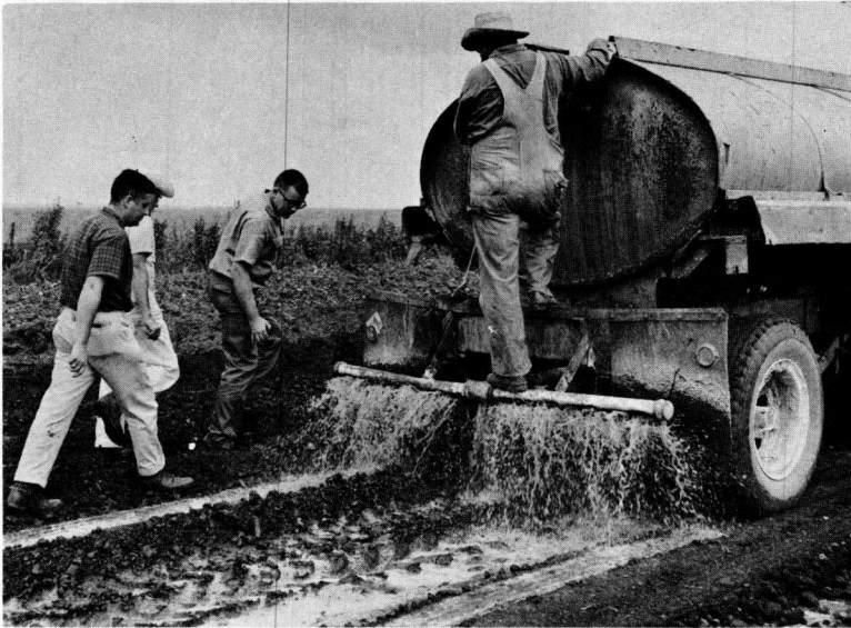
Figure 16. Aliquat H226 solution being applied to road from water distributor.
