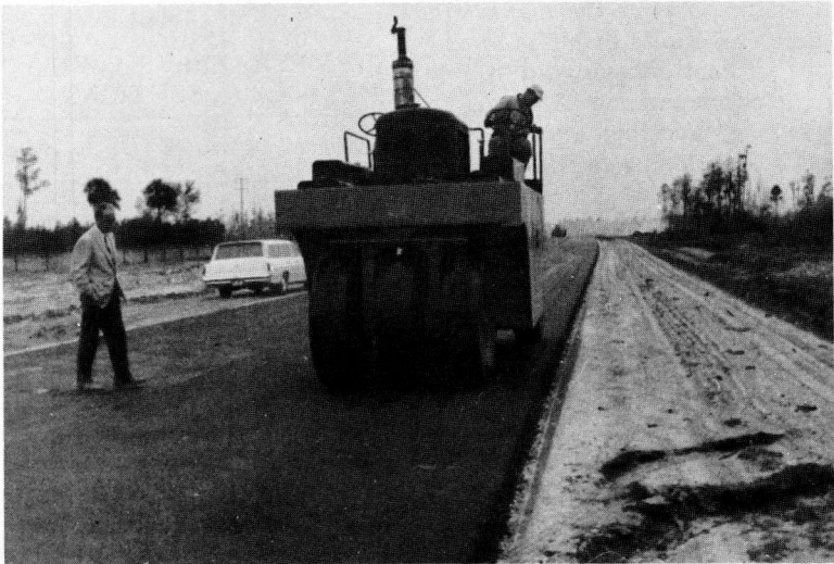
Figure 6. Bros SP-730B pneumatic-tired roller in operation.
