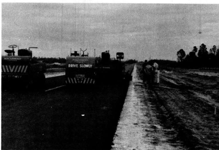
Figure 5. Barber Greene spreader, 5-ton tandem wheel roller, and Bros SP-54B pneumatic-tired roller parked between test sections during break in construction operations.
