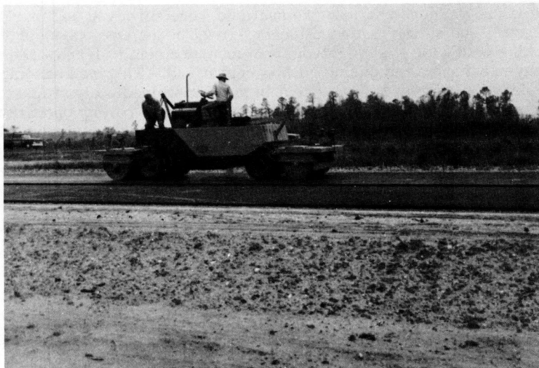
Figure 7. Vibratory roller in operation.
