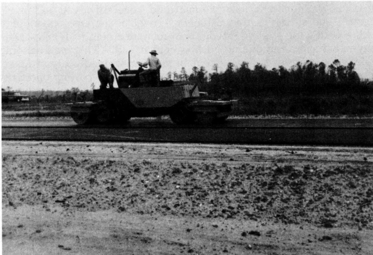
Figure 7. Vibratory roller in operation.
