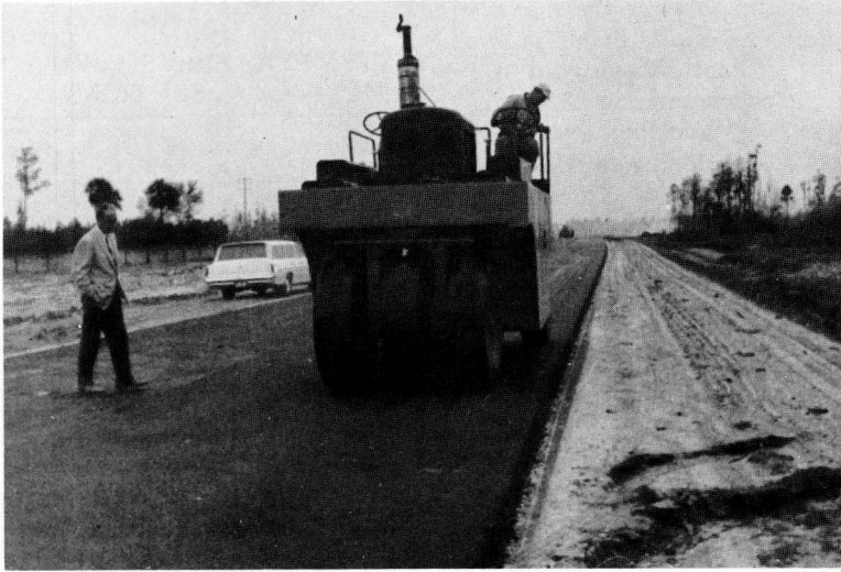
Figure 6. Bros SP-730B pneumatic-tired roller in operation.
