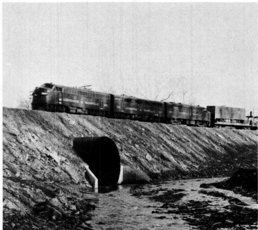
Figure 30. A 20-ft diameter, 1 gage MULTI-PLATE culvert under mainline of L&N RR near Independence, Ky.
