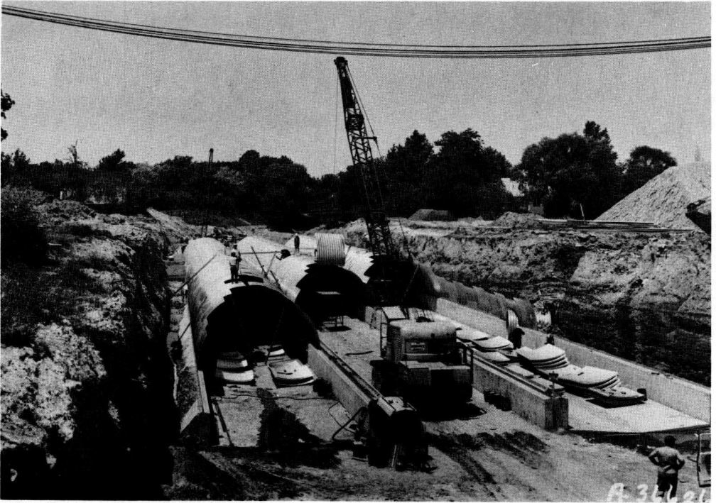
Figure 33. Triple 20- by 10-ft MULTI-PLATE Arch located under Interstate 90 in Cleveland, Ohio. Maximum fill on this 1,000-ft long culvert is 20 ft, yet deflection is practically negligible.
