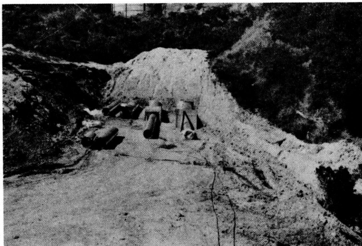
Figure 1. General view of test site showing pipe runs in approximate position.
