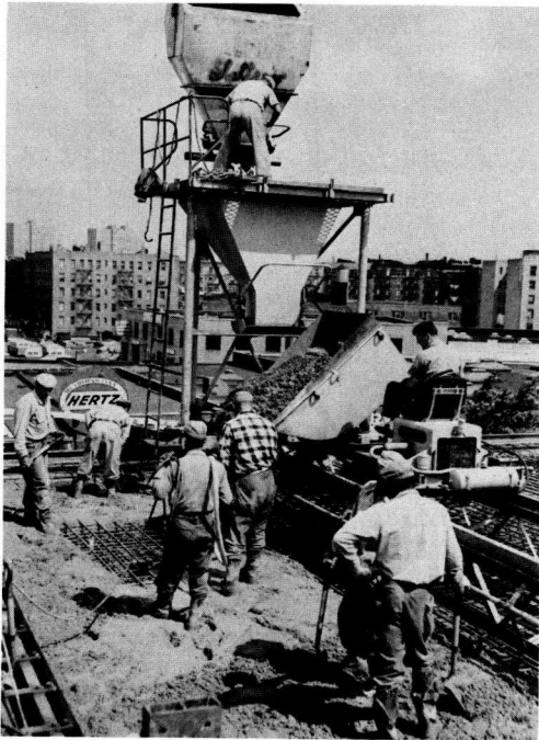
Figure 2. Deck under construction.
