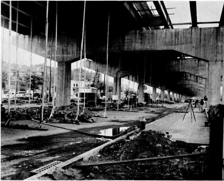
Figure 3. Bridge during construction.
