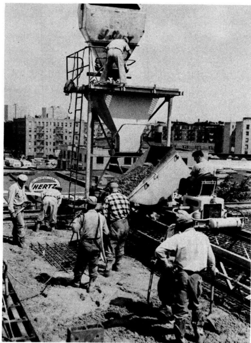
Figure 2. Deck under construction.
