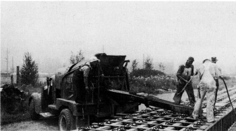
Figure 9. Placing Concrete in Stringers
