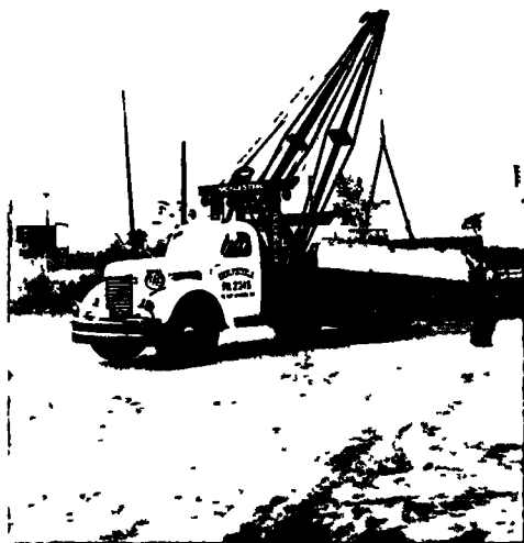
Figure 10. Baker River Bridge - Handling Precast Stringers with Towing Truck
