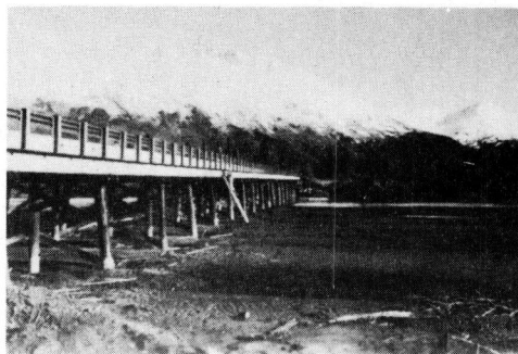
Figure 5. Placer River Bridge, Alaska - Perspective of Completed Trestle
