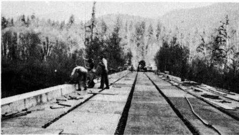
Figure 16. Baker River Bridge - All Precast Stringers and Panels in Position Ready for Filling of Joints
