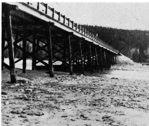
Figure 6. View of Kenai River Bridge, Kenai Peninsula, Alaska - Stringers for Deck Precast
