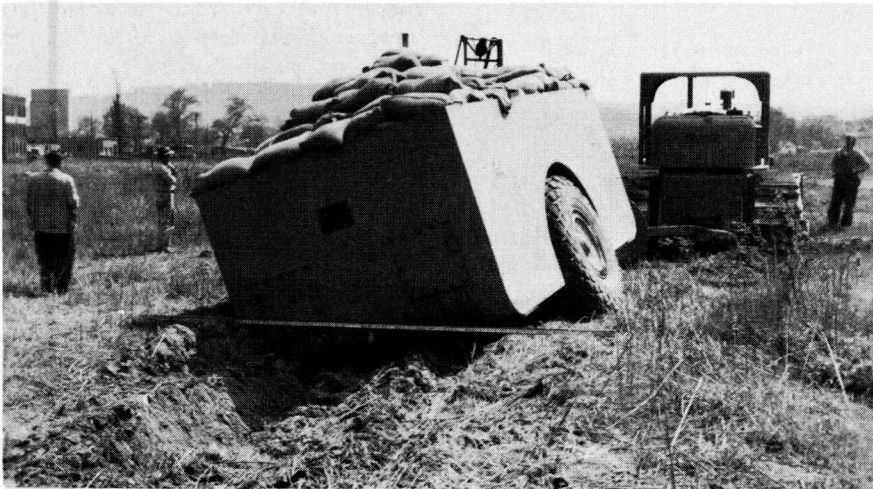
Figure 9. Test Strip 7 Showing 50-Ton Roller Boggling Down During First Pass. No Prior Rolling given.
