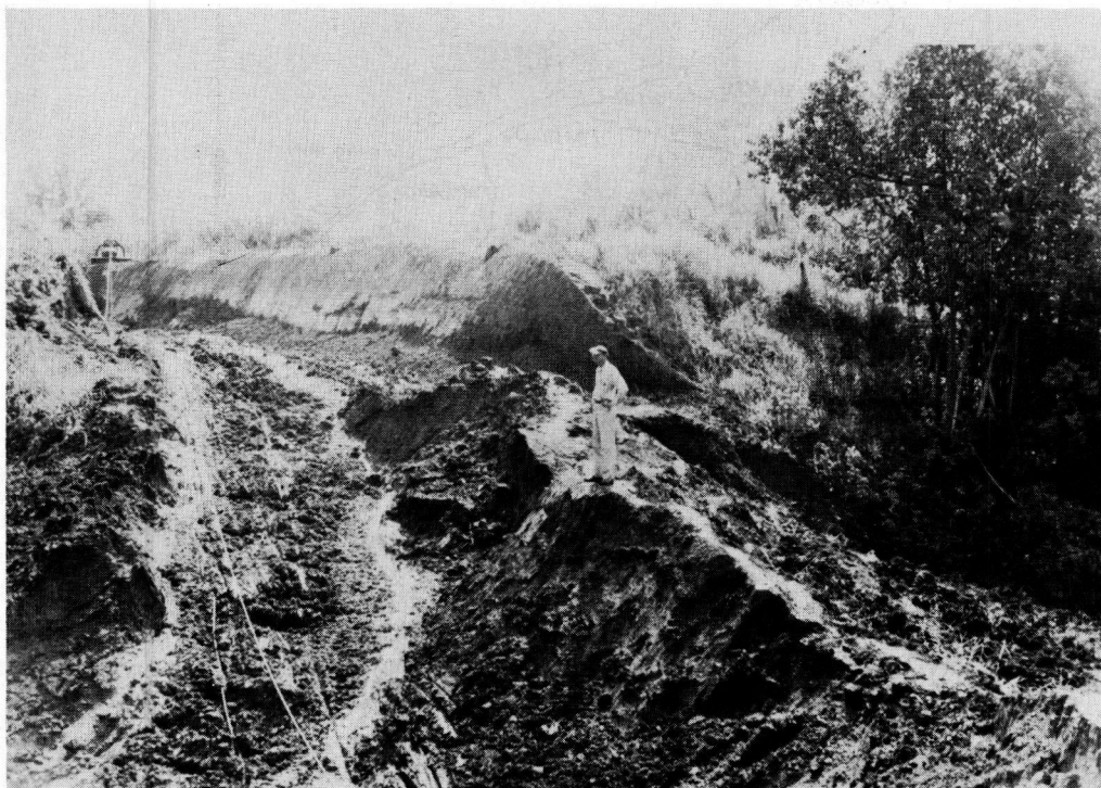
Figure 2. Embankment Slide Due to Intensive Working of Material Using a Sauerman Bucket. Note contrasting stability of cut slopes in background.
