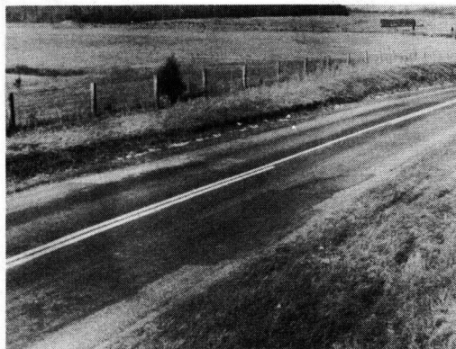
Figure 22. Performance of pavement in an area of Iredell. Failures always occur on B-horizon; none on C-horizon.
