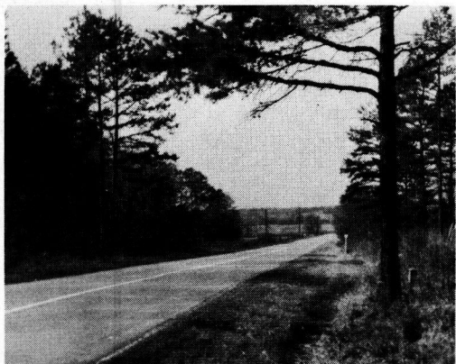
Figure 26. Flat terrain of Wadesboro soils. Wet subgrade has caused the rutting which is evidenced by a wavy centerline.
