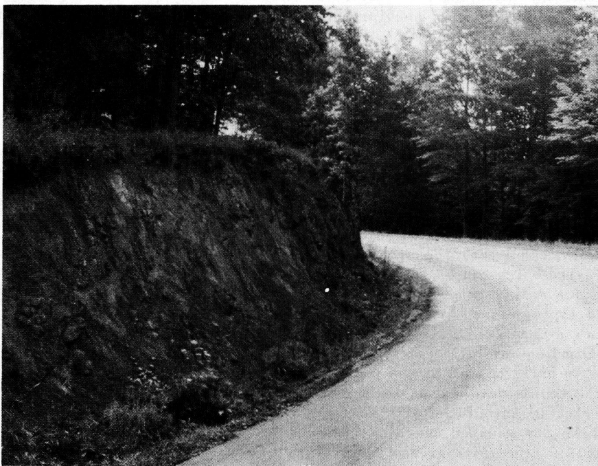
Figure 4. Soft weathered rock exposed in the profile of the Lloyd Soil Series. Poor surface drainage and clay-like soils caused the edge failure in the curve.
