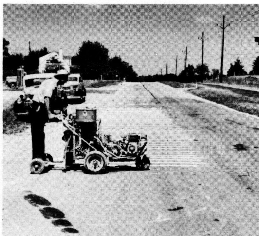
Figure 1. 1950 Transverse stripe location. Stripes on bituminous surface are immediately behind striper and on concrete surface in the background.
