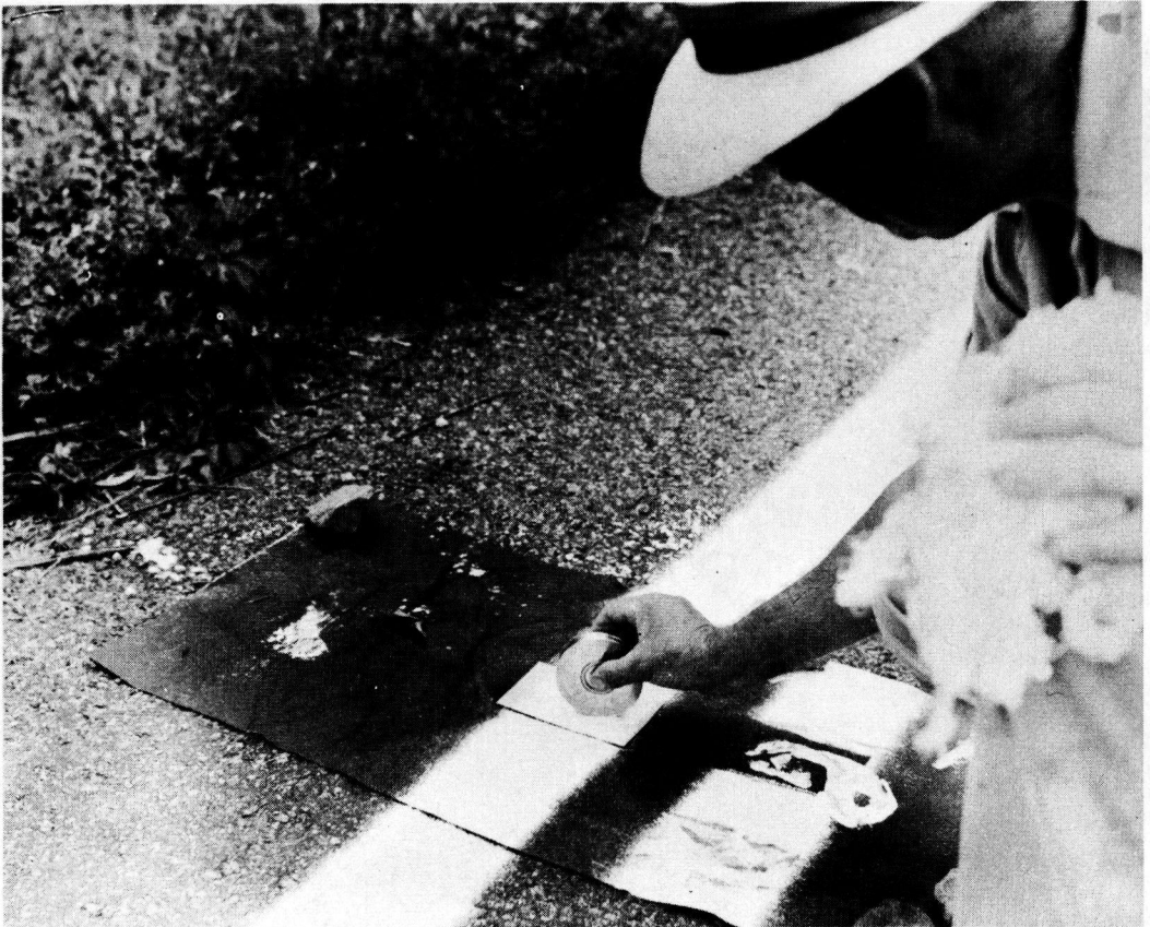
Figure 3. Wet-film-thickness gauge in use.
