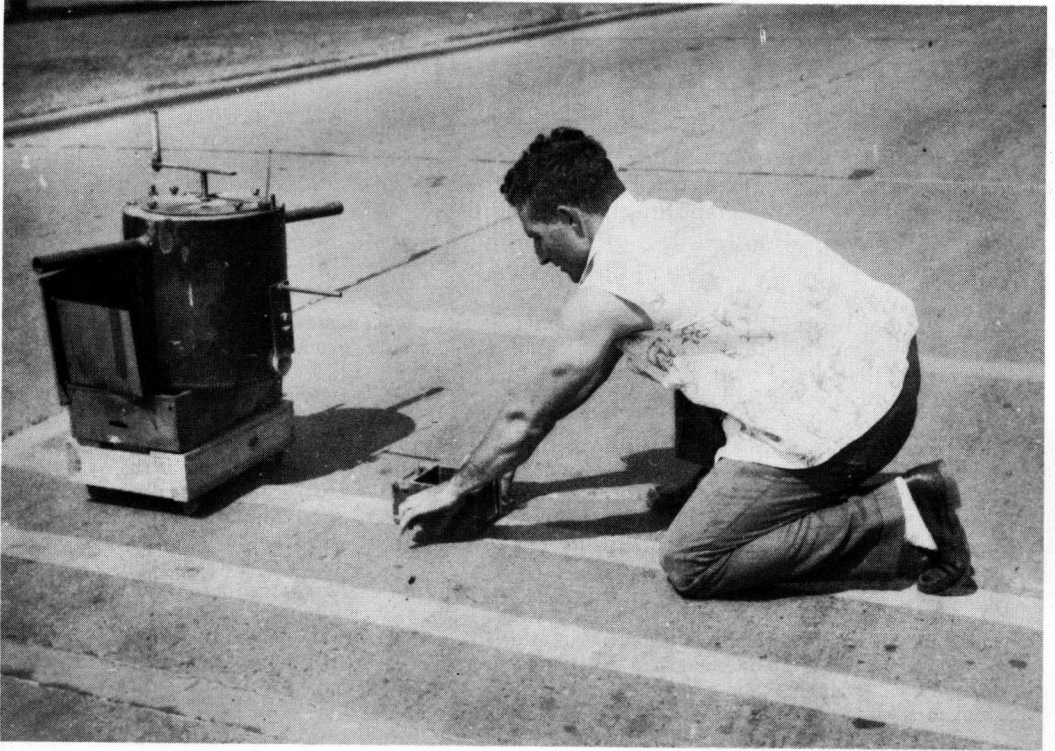
Figure 1. Laying rosin striping compound.
