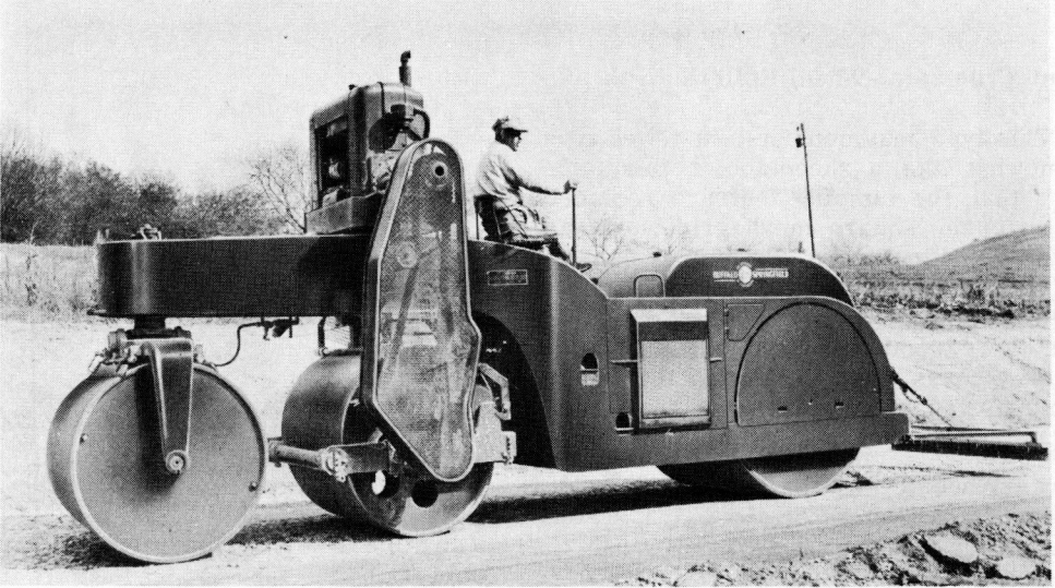
Figure 28. Tandem roller with vibratory intermediate roll.
