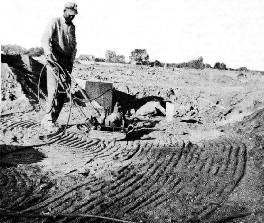
Figure 29. Small, hand-operated self-propelled, vibrating-baseplate compactor.
