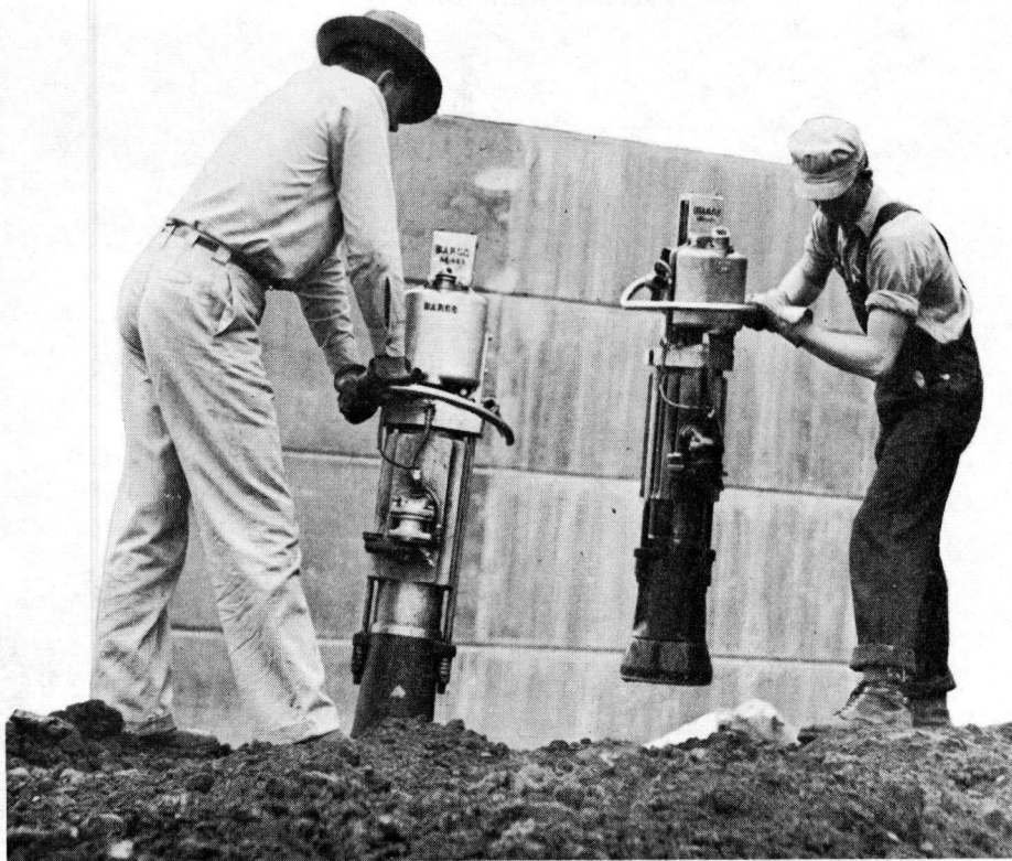
Figure 33. Gasoline-driven rammers for compacting soil in restricted areas.
