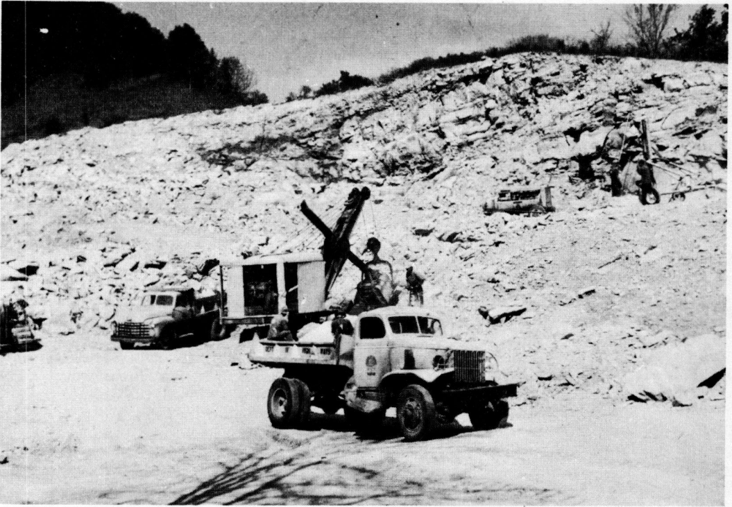
Figure 6. Quarrying Pennsylvanian sandstone for construction of a bituminous test pavement on Kentucky Route 30. Unusual variations in the form and quality of sandstone deposits constitute problems in materials surveying.
