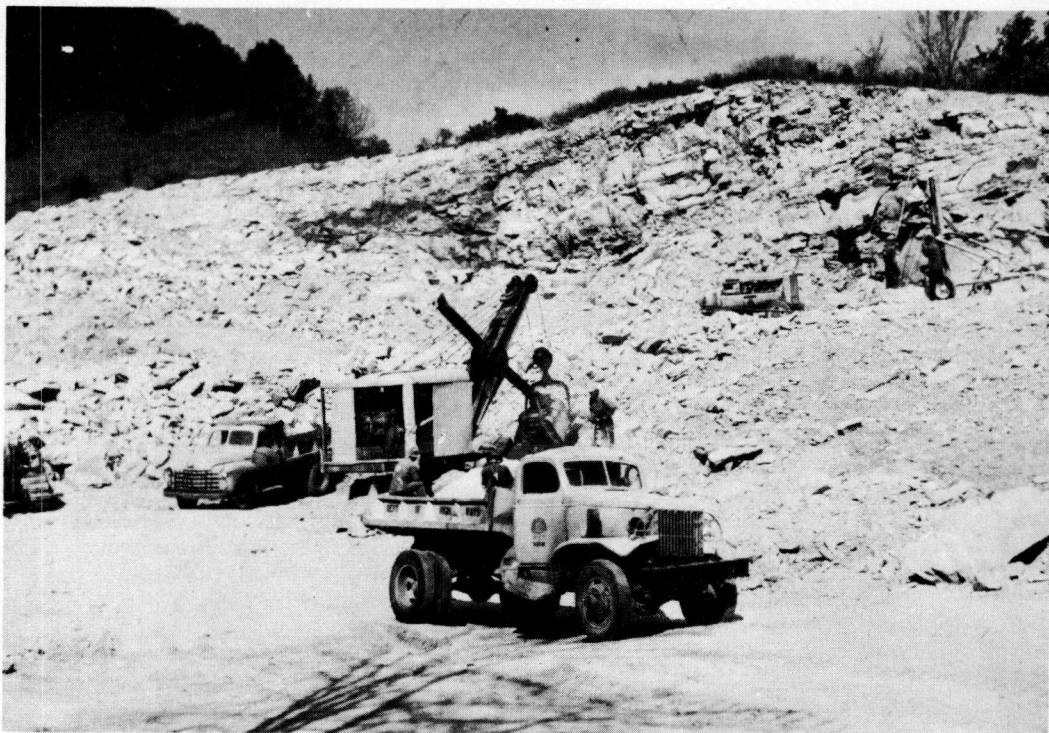
Figure 6. Quarrying Pennsylvanian sandstone for construction of a bituminous test pavement on Kentucky Route 30. Unusual variations in the form and quality of sandstone deposits constitute problems in materials surveying.
