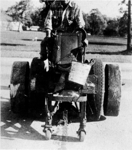
Figure 10. This garden-type tractor with concrete weights was used on two of the 1961 contracts for the cleaning of tranverse joints. The pail shown hanging from the tractor was used for carrying extra cutters and tools.
