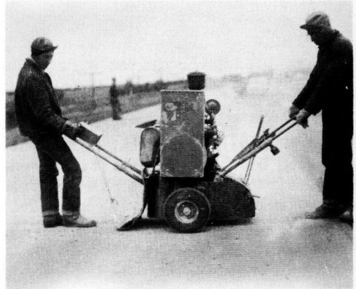
Figure 17. Concrete-grooving-and-joint-cleaning machine used for cutting cracks.
