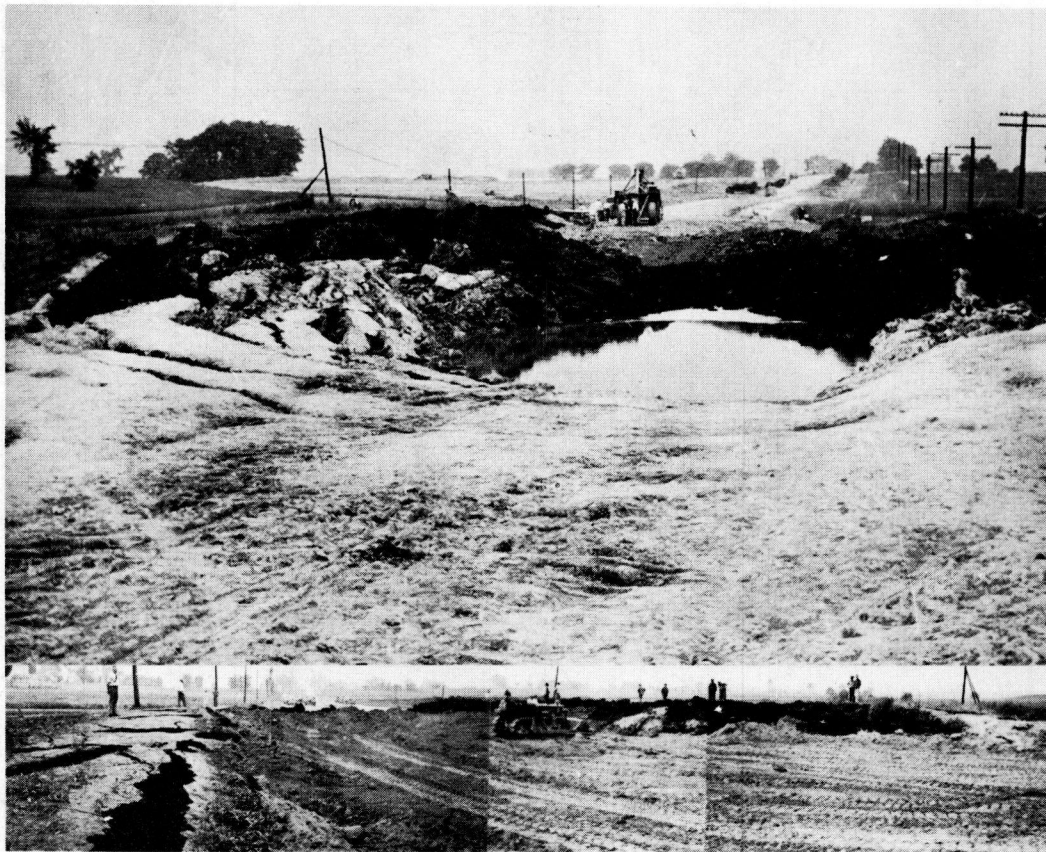
Figure 6. Peat bog, Wisconsin Glacial Drift. S.R. 18, Lorain County, Ohio. The peat is being displaced by loading. Note upheaved peat at left and right of the lower photograph.
