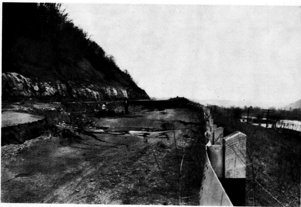
Figure 7. Landslide, Conemaugh Formation Pennsylvania Series S.R. 7, Lawrence County, Ohio. This slide developed after construction of a side-hill fill on sloping talus. Correction consisted of loading the toe of the slide and adding fill at the top together with improvement of the surface drainage.
