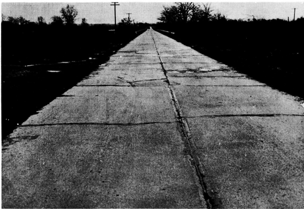
Figure 9. Pumping and broken concrete pavement on Route 30N, Crawford County, Ohio. A 9-7-7-9 concrete pavement on till plain clay of late Wisconsin Age; no subbase.
