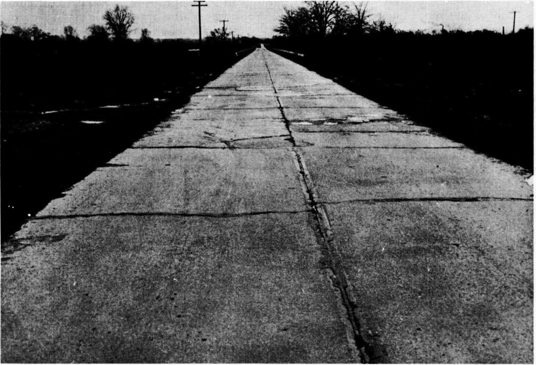
Figure 9. Pumping and broken concrete pavement on Route 30N, Crawford County, Ohio. A 9-7-7-9 concrete pavement on till plain clay of late Wisconsin Age; no subbase.
