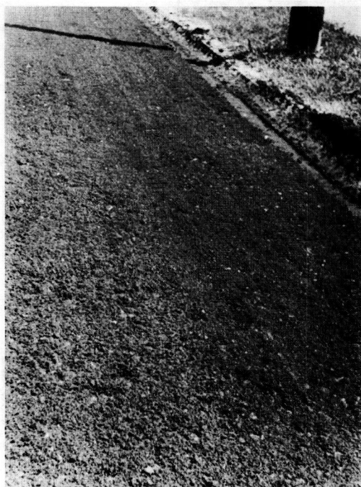
Figure 13. Condition of road base prior to compaction and after mixing lime and flyash into the soil, HiNella, N. J.
