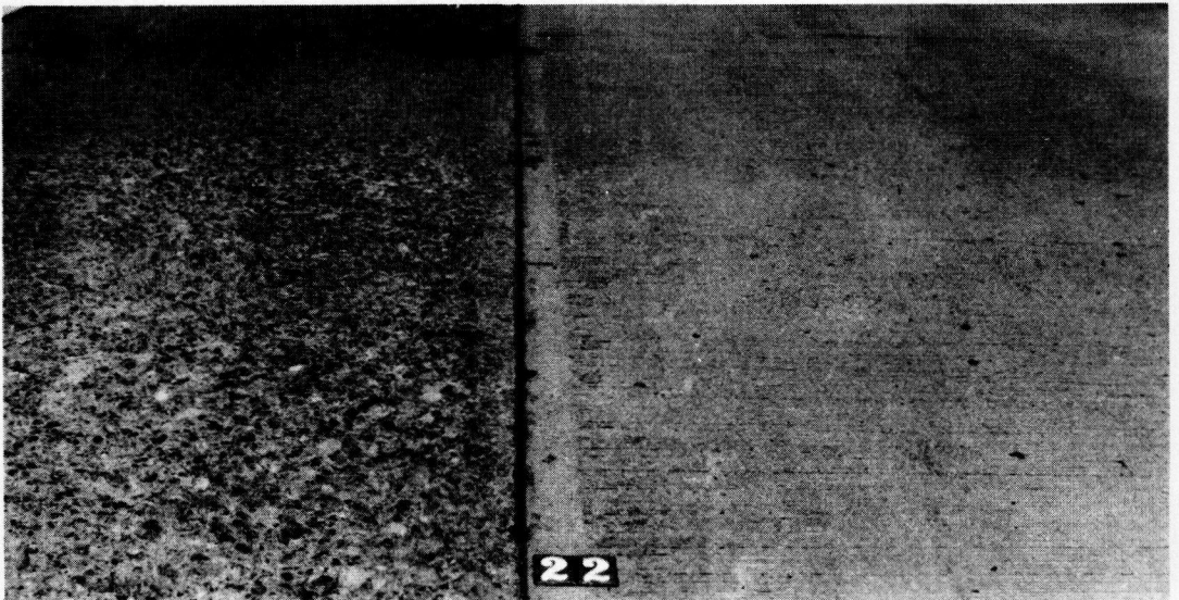
Figure 3. Route 30, Hope Center-Wells, New York, Station 578 + 00.
