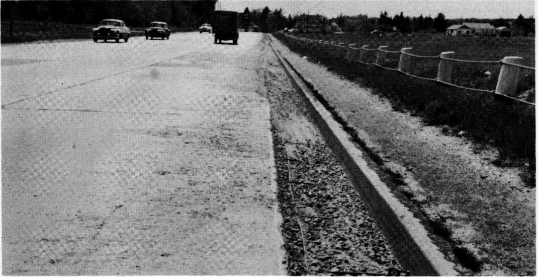
Figure 8. US 1, Scarborough, Maine, Station 243 + 30.
