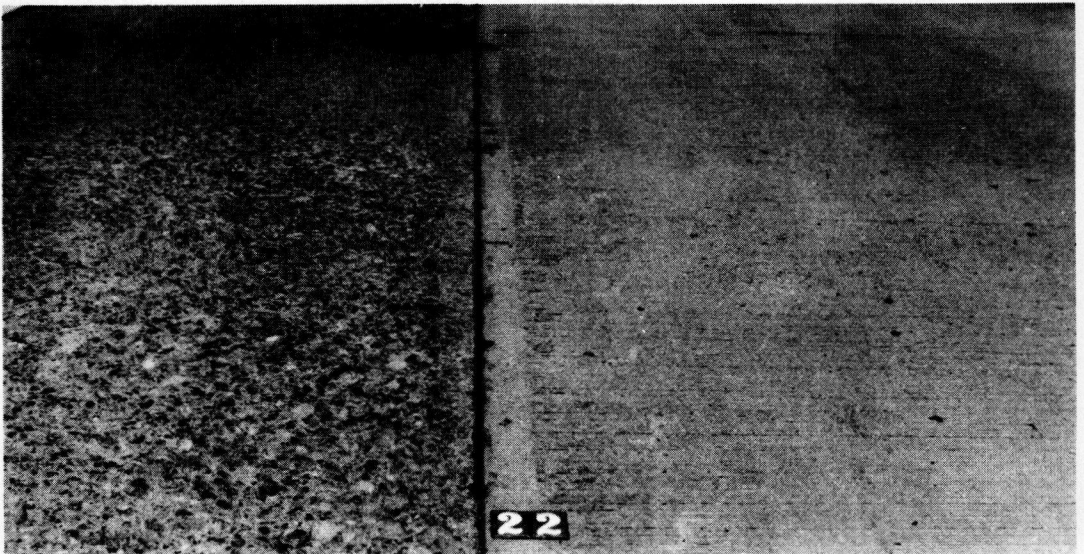
Figure 3. Route 30, Hope Center-Wells, New York, Station 578 + 00.
