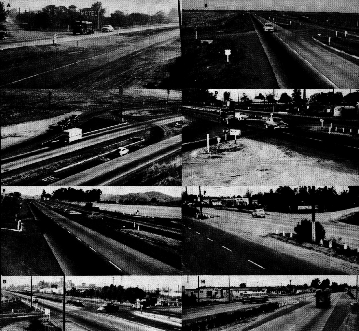
Figure 4. Typical intersection types: (A) Intersection 105, uncurbed crossover; (B) Intersection 146, curbed crossover; (C) Intersection 159, curbed and channelized; (D) Intersection 65, an older design; (E) Intersection 160, a recent design type; (F) Intersection 112, a very-low-volume T intersection; (G) Intersection 75, crossroad count is 2,500 vehicles per day; and (H) Intersection 116, old traveled way used as frontage road.
