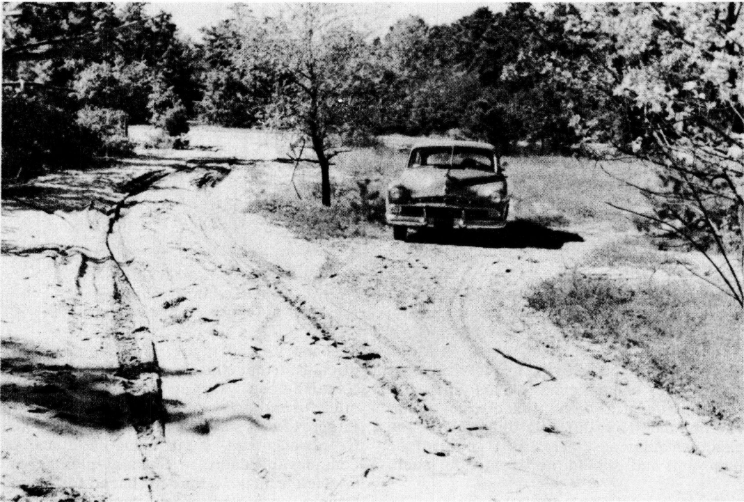
Figure 15. A bypass and rutting on forest road. This rutted sandy soil in left hand portion of photograph will discourage further traffic. Automobile is leaving newly formed bypass at right.
