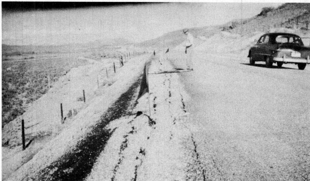
Figure 9(b). Ground view of cracking and subsidence adjacent to the higher and steeper fill-slopes, due to excessive spring runoff, on a highway constructed along alignment in Figure 9(a).
