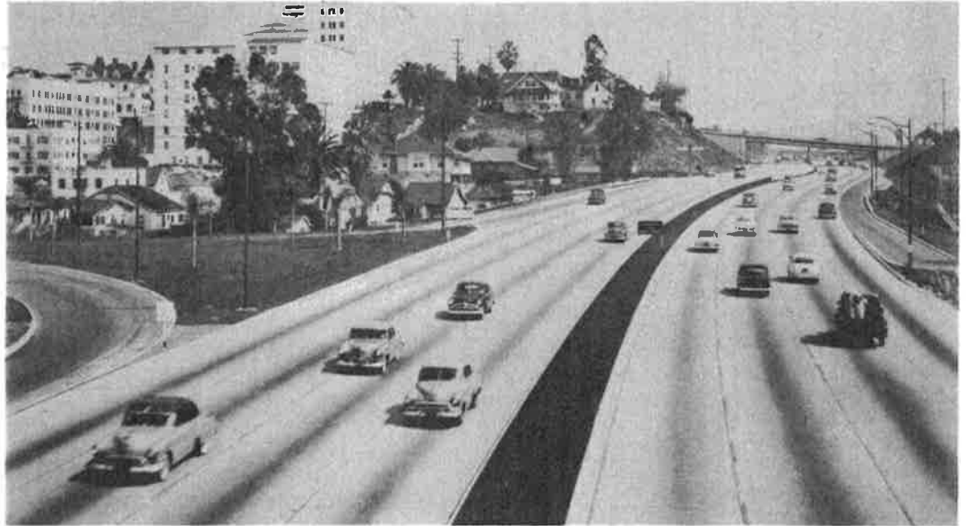
Figure 9. Hollywood Freeway in Los Angeles.
