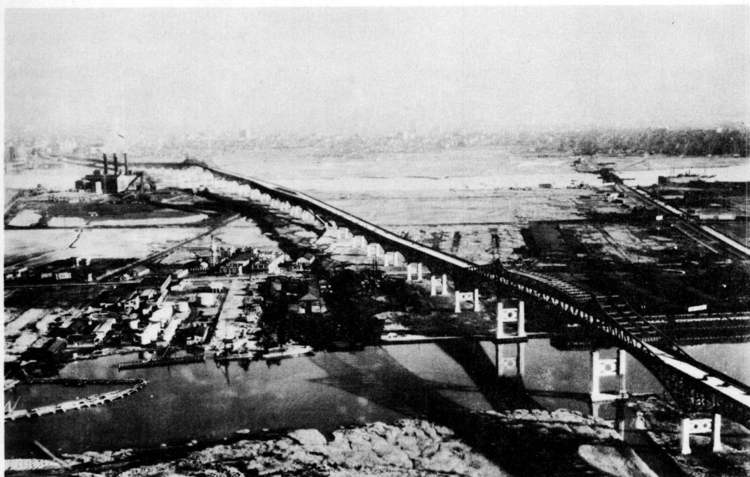
Figure 5. Pulaski Skyway, an example of a high-level viaduct.
