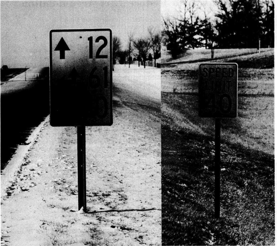
Figure 1. Normal dirt accumulation on typical rural signs 4 feet up and 6 feet from pavement edge.
