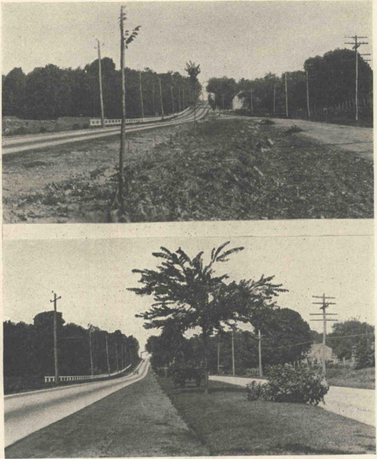
Figure 5. The upper view shows the unsightly island area created at the time the new concrete road was constructed in the Town of Montville, Conn., and the old roadbed abandoned. The after effect may be appreciated in the lower picture of the same location.
