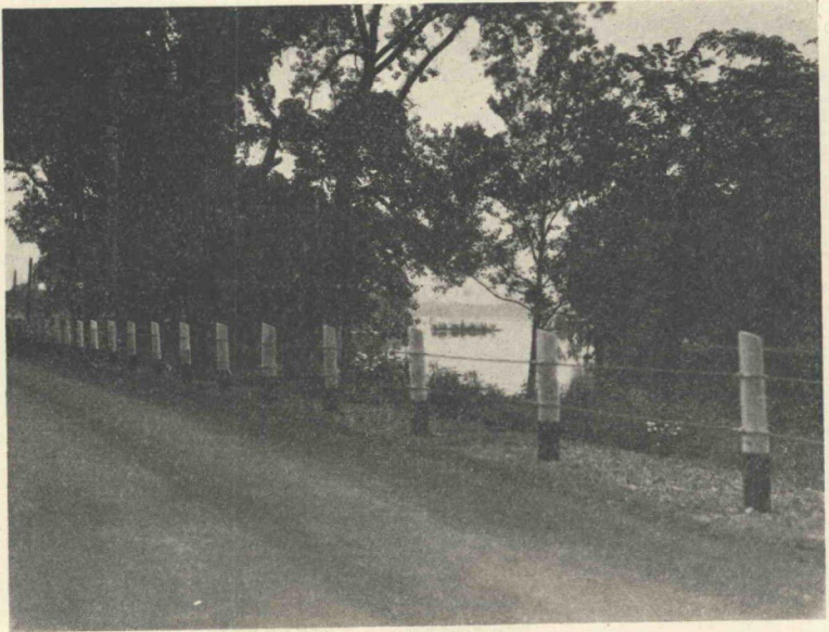
Figure 1. This picture illustrates the method used by the Connecticut Highway Department in opening up vistas adjacent to rivers in which it is the policy to offer to the motorist frequent glimpses of the water rather than one continual panorama.
