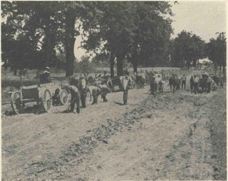
Figure 7. Typical View Showing Road Under Construction
