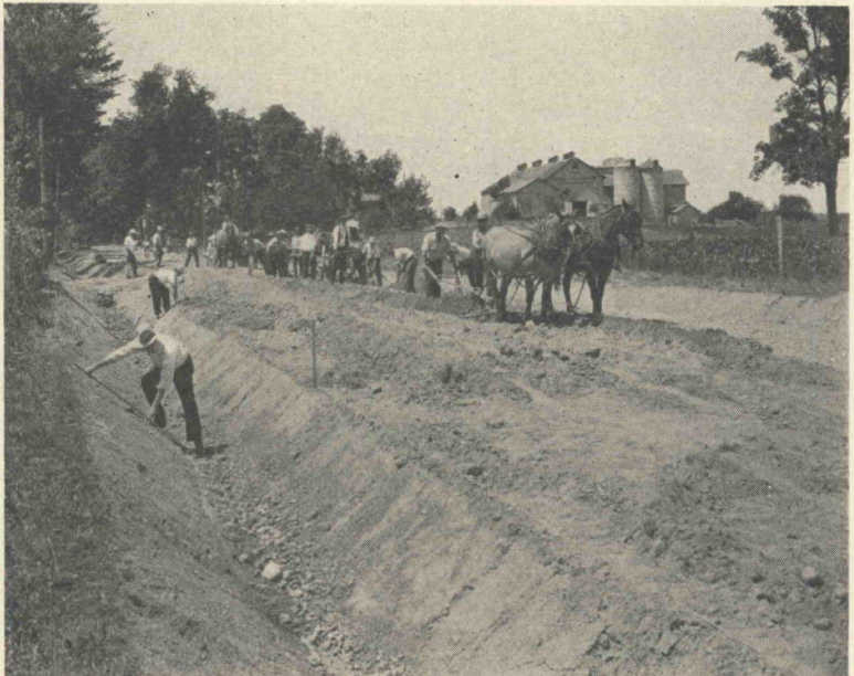
Figure 8. Typical View Showing Road Under Construction
