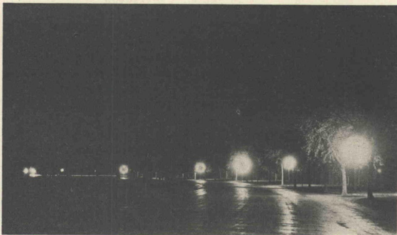
Figure 2. Inefficient Light Application. 10,000-Lumen lamps—13-Ft. Mounting Height. 173-Ft. Linear Spacing. Lamps 3 ft. back of road surface. Asphalt Pavement. Note how specular reflection does not cover traveled road surface. Lighting conditions would be even worse than indicated on a straight-away.
