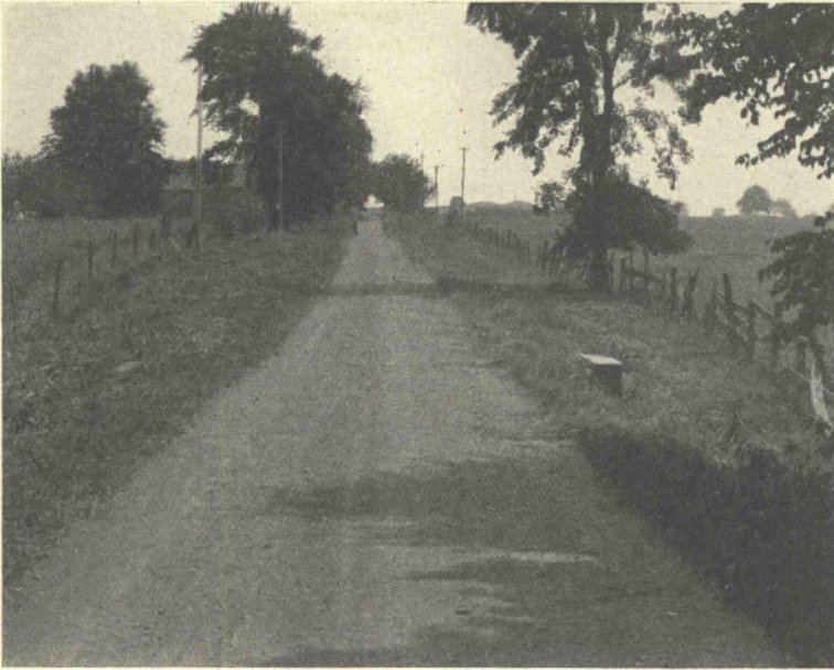
Figure 5. Road before Start of Construction
