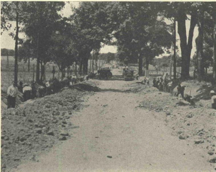
Figure 6. Road Under Construction
