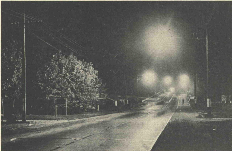
Figure 7. Most Effective Equipment Placed in Most Effective Manner Reveals Pedestrian or Object on Road by Silhouette.
