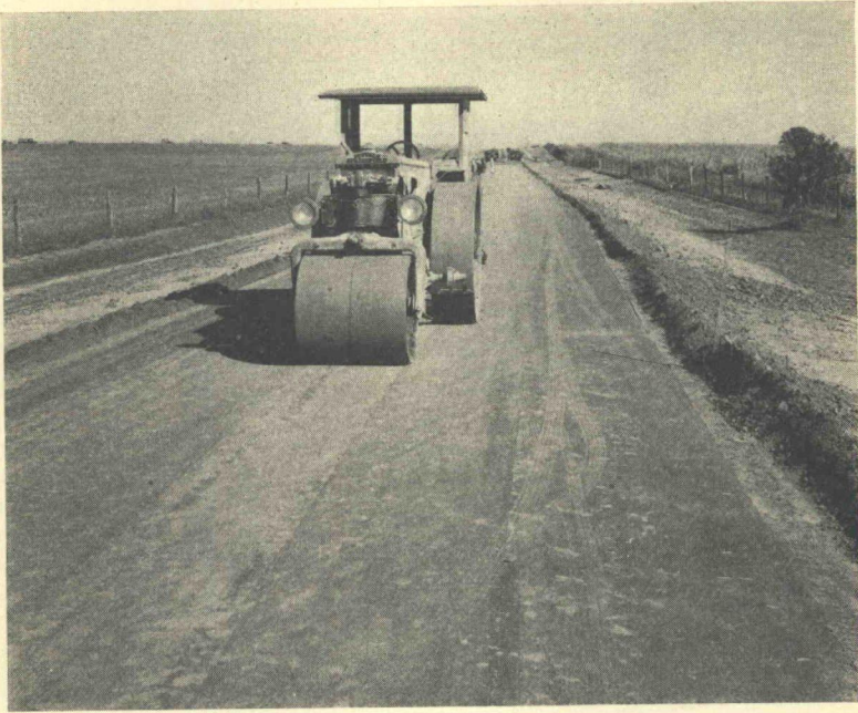
Figure 19. Final compaction with an 8-ton three wheel roller. Illinois photo.
