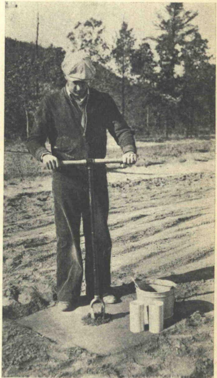
Figure 3. Drilling hole for determining density of hardened road.
