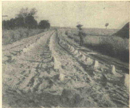
Figure 3. Cement sacks were placed at a specified rate and emptied prior to spreading with a motor grader. Missouri photo.
