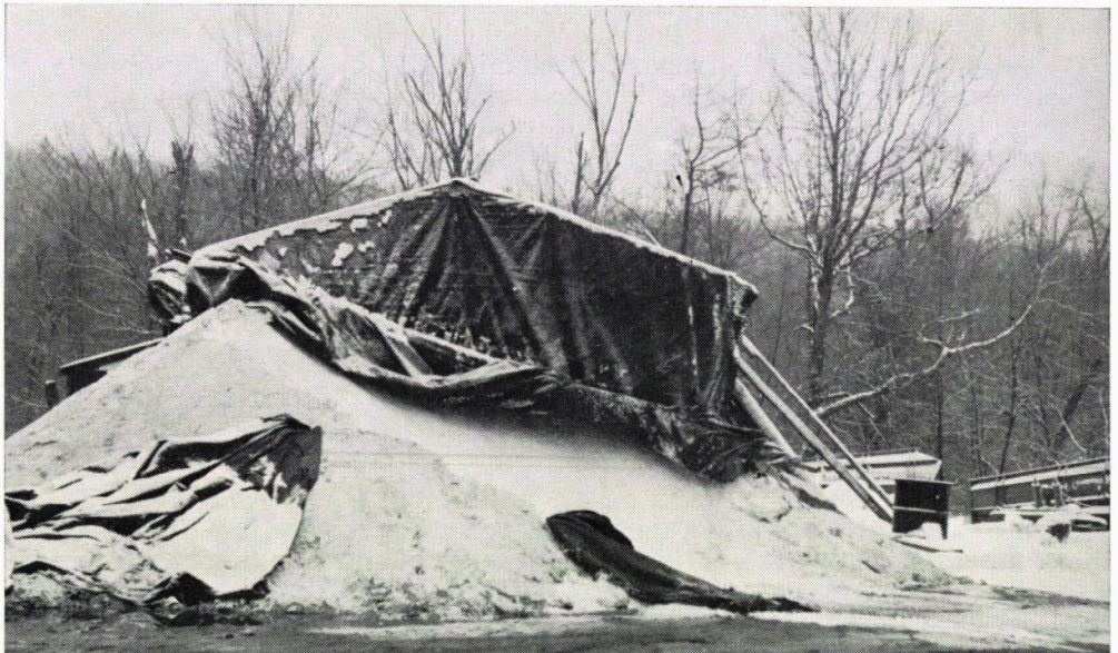
Figure 1. Calcium chloride storage shed with surplus stored outside.
