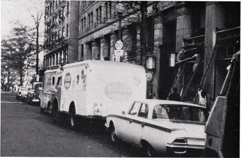
Figure 4. Advance turn marker installation largely hidden from view of approaching driver by truck on extreme right.
