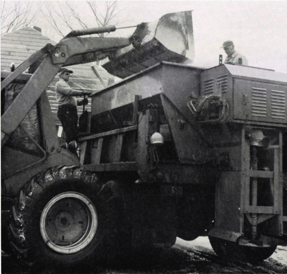
Figure 2. Loading demountable sander with mixture.
