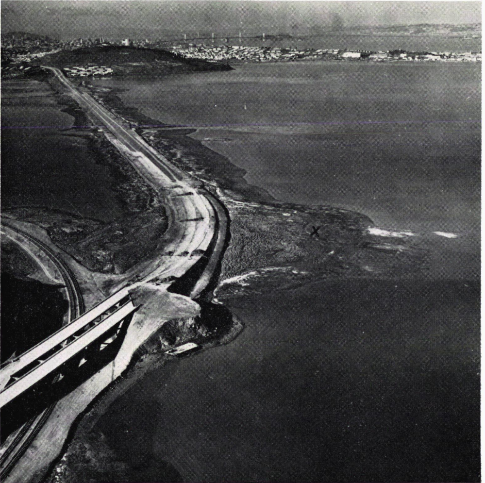
Figure 1. General view of open water fill, final grading operations in progress.
