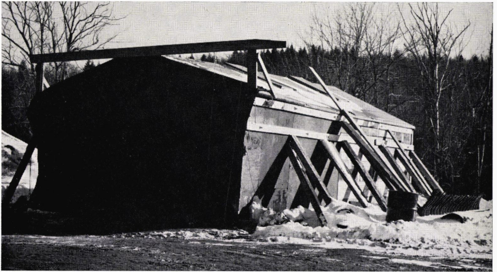
Figure 3. Calcium chloride storage shed closed by tarpaulin between storms.
