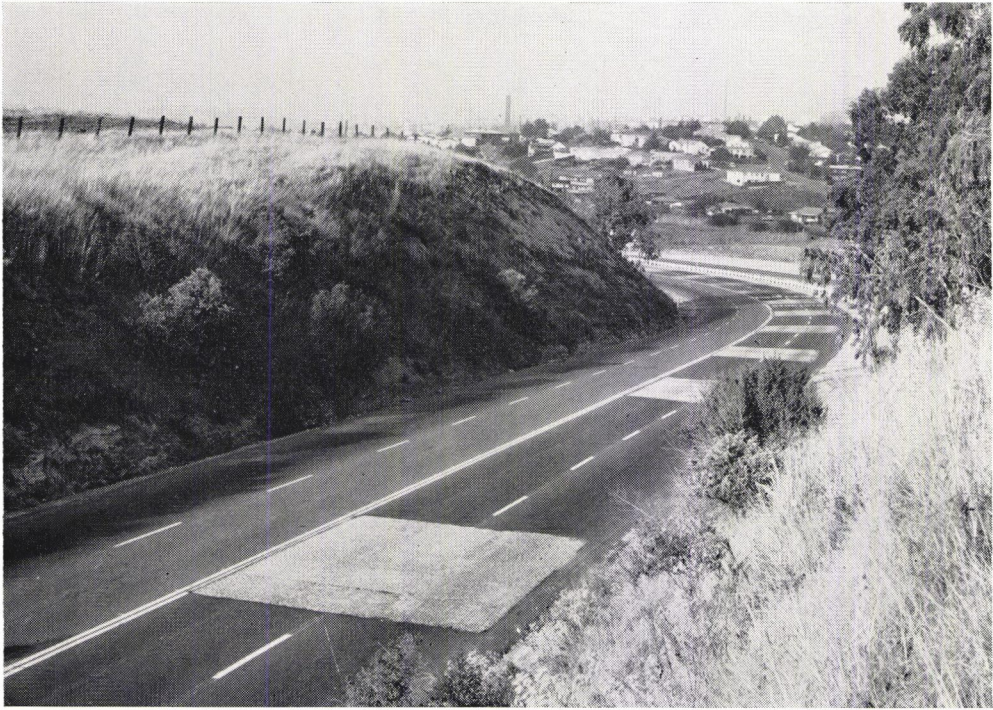
Figure 6. Appearance of rumble strip experiments on old US 40, Case III.
