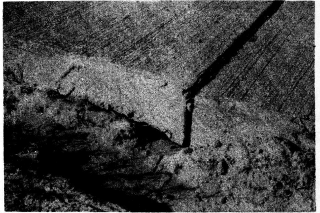
FIGURE 14. SEVERE PUMPING AT AN UNTREATED JOINT IN THE SECTION OF PAVEMENT IN WHICH JOINTS WERE TREATED WITH MIX "A"
